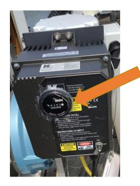
We use the GPM and your unit's hour meter reading to approximate how many gallons of sewage your unit has pumped over the last year.
