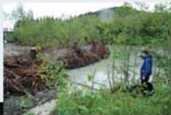
Mendenhall River Engineered Log Jam, Juneau, AK
