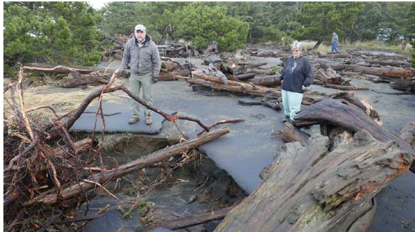
The Jan. 18, 2018 storm wreaked havoc on campsites and structures at Cape Disappointment State Park. An entire loop of campsites was closed indefinitely in 2018 due to erosion from this and other storms
