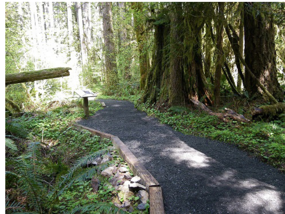
The trail material can be compacted gravel
